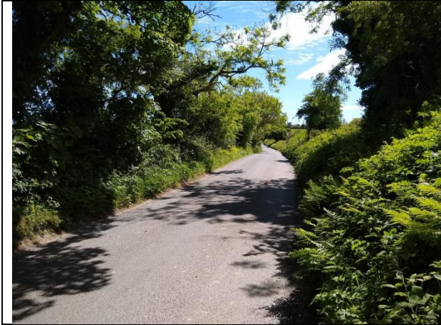
Plate 3. View south, well-developed hedgerow and treeline on both road verges. Eastern (left of image) hedgerow / treeline to be removed.
